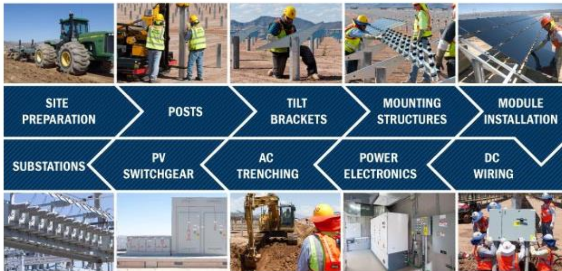
Figure 4: Illustration summarising the construction of a typical Solar PV Power Plant (Source: Solar DAO, 2020)
